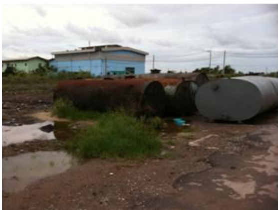
Figure 1 petroleum hydrocarbon storage tanks and leakages to surrounding area.
