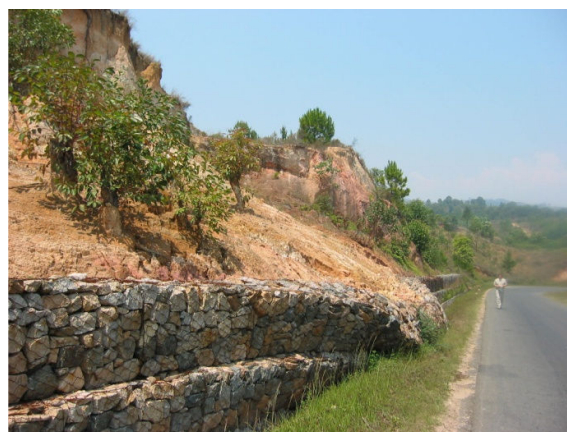
Figure 10 Madagascar: stabilization of slope with gabions. Though not fully successful in this case, the measure is usually effective and one of the most inexpensive and most widely used methods for road slope stabilization in developing countries (Photo NGI)
