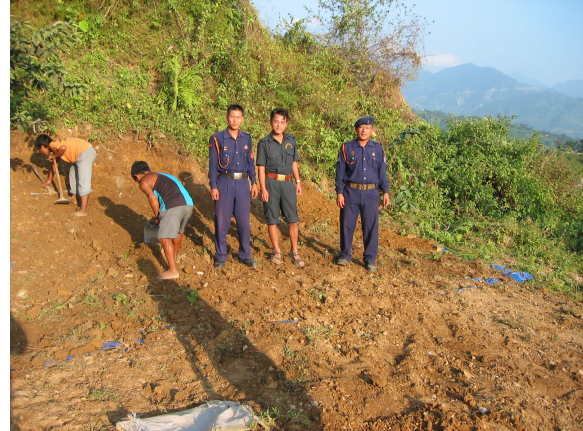
Figure 16: Placement of plastic sheet on the tension cracks and covering with soil
