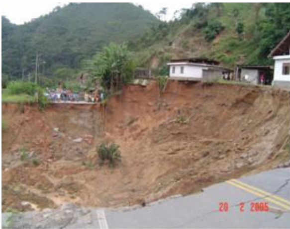
Figure 6 Brazil, Road in the vicinity of Rio de Janeiro that collapsed due to a rainfall triggered landslide in 2005, isolating a small neighbouring town (Photo F. Bogossian)
