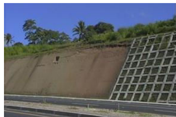
Figure 13: El Salvador: road cut stabilization with anchored concrete ribs and large open net- protected weep holes (Photos University of El Salvador)
