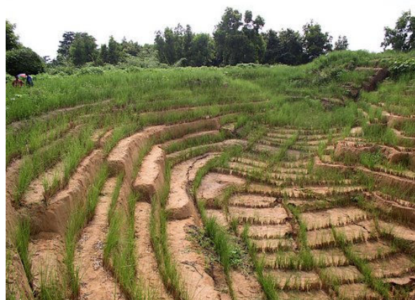
Figure 11 This planting of Vetiver grass is about 3 month old. Vetiver grass has shown to be an effective means of stabilization at a low cost in many countries (L. Highland,USGS)
