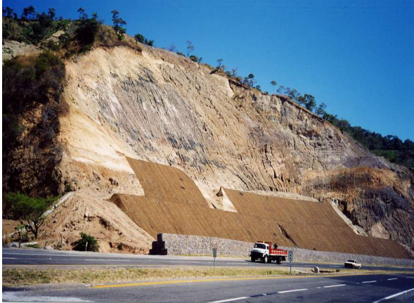
Figure 12. El Salvador: Rehabilitation of the La Leona Landslide where erosion protection of the new slope made use of coca mats (Photo Servicio Nacional de Estudios Territoriales (SNET))
