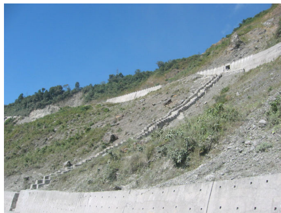
Figure 9 Bhutan: surface water system for stabilizing the road in an unstable slope that has experienced movements over many years (Photo NGI)
