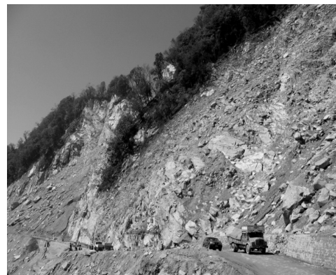
Figure 4: Bhutan: the highway between Thimpu and Phuentsholing experiences severe landslides in most monsoon periods and was closed for 3 months in 2001 due to complete blockage (Photo NGI, Bhasin et al. 2009)
