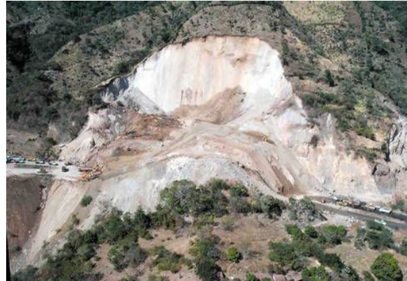
Figure 8 El Salvador: Blocking of the Pan American Highway at La Leona from a landslide caused by the 2001 Earthquake of Magnitude 7.6 (Photo Servicio Nacional de Estudios Territoriales (SNET))
