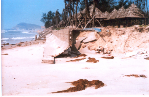
Photo 1 Collapse sea-wall in Thuy Duong resort due to erosion
